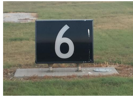
Figure 10: Runway Distance Remaining sign
