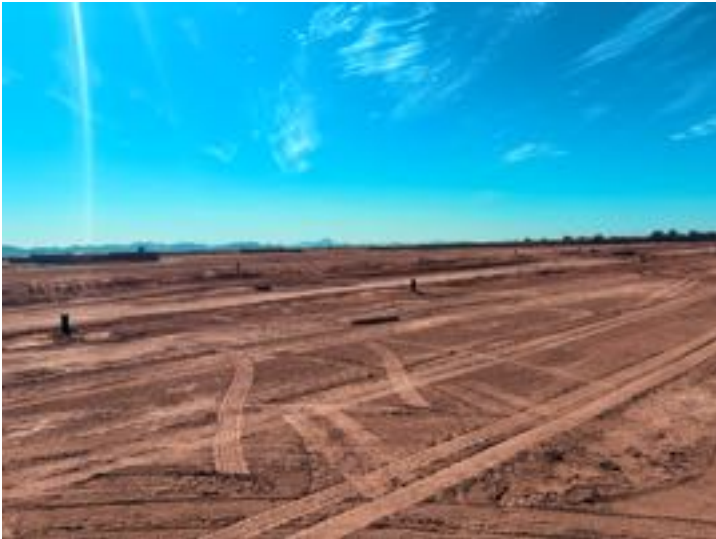
9– Looking southwest across 7s and 8.
