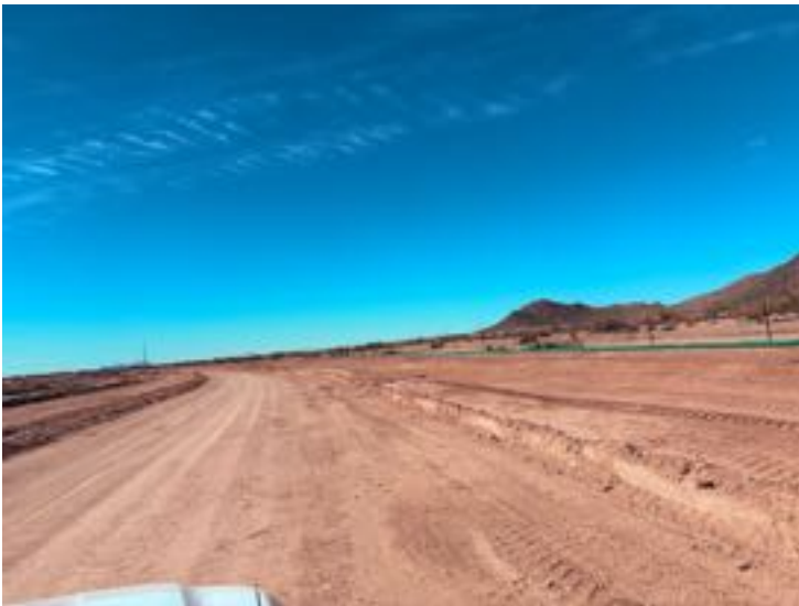
11 – Looking west along Westpark Loop North.
