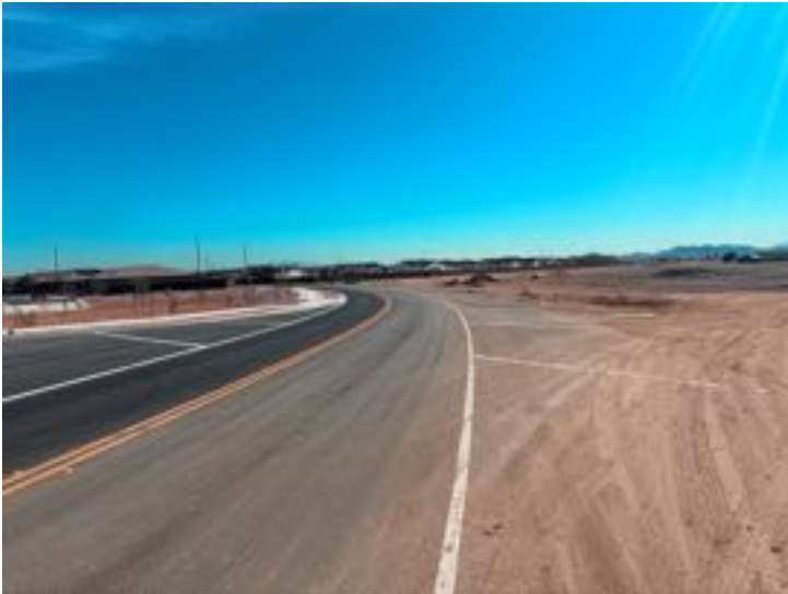
2 – Looking south along Westpark Loop.
