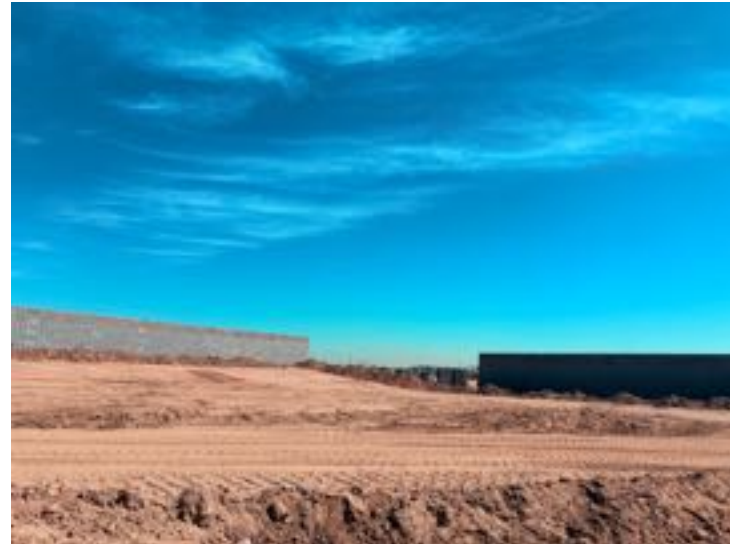
4 – Looking east across Parcel 20N.
