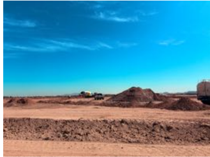
10 – Looking south along 7S and 8.
